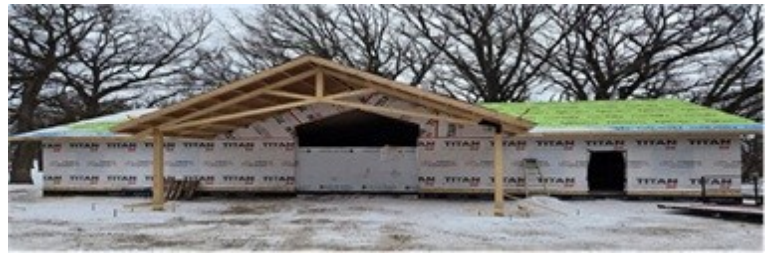
New Cabin is Coming Along!
